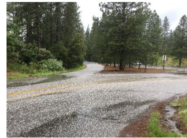
A free right turn lane from SR 49 onto W Broad Street allows for high-speed turns
