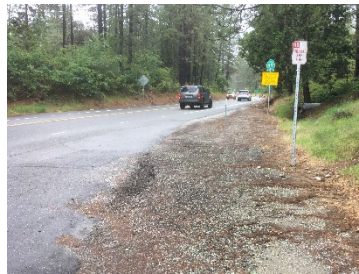
No facilities are provided for people walking or bicycling along SR 49, and curves in the roadway create sight distance challenges
